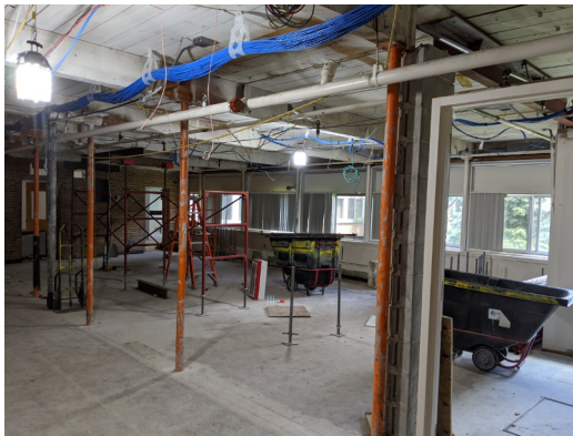
Sheridan Hills – C wing progress. SPED area underground plumbing rough-in. Level 2 Classroom above ceiling rough-in and plumbing wall framing.
