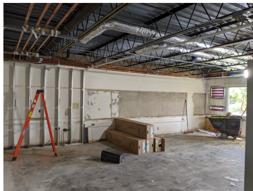
Sheridan Hills – C wing progress. SPED area underground plumbing rough-in. Level 2 Classroom above ceiling rough-in and plumbing wall framing.
