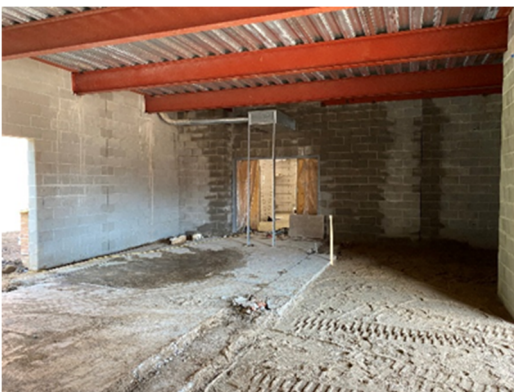
High School – Area P Link Cabinet Unit Heater Installation, Roof and Window Wood Blocking
