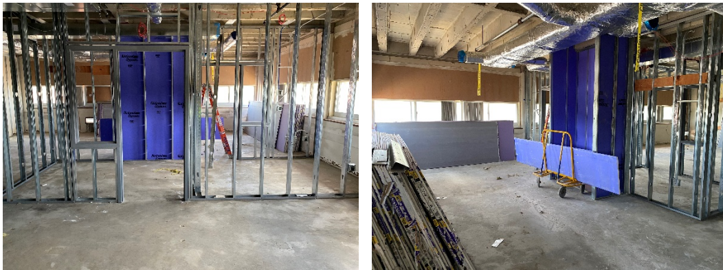
Middle School – Third Floor Resource Area Wall and Soffit Framing
