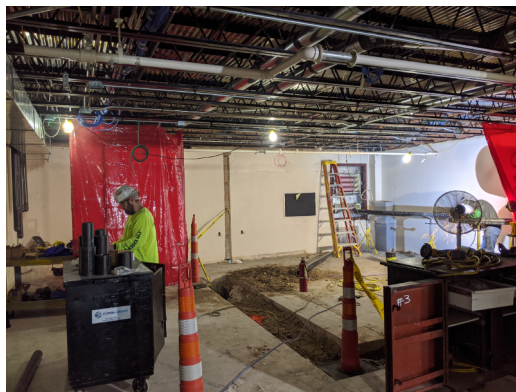
Sheridan Hills – C wing progress. SPED area underground plumbing rough-in. Level 2 Classroom above ceiling rough-in and plumbing wall framing.
