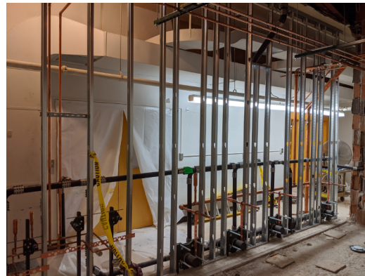
Sheridan Hills – C wing progress. SPED area underground plumbing rough-in. Level 2 Classroom above ceiling rough-in and plumbing wall framing.
