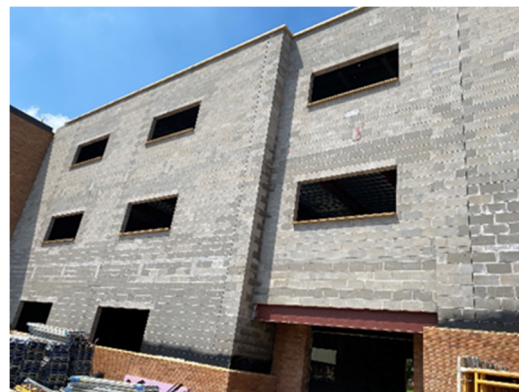
High School – Area P Link Cabinet Unit Heater Installation, Roof and Window Wood Blocking
