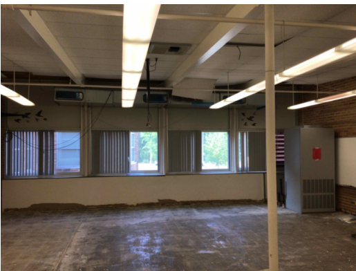
Sheridan Hills – Duct work and unit ventilator installation in the classrooms.
