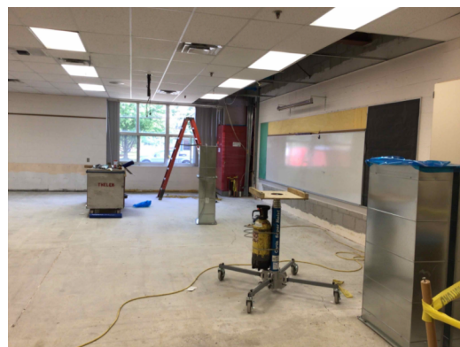
Sheridan Hills – Duct work and unit ventilator installation in the classrooms.
