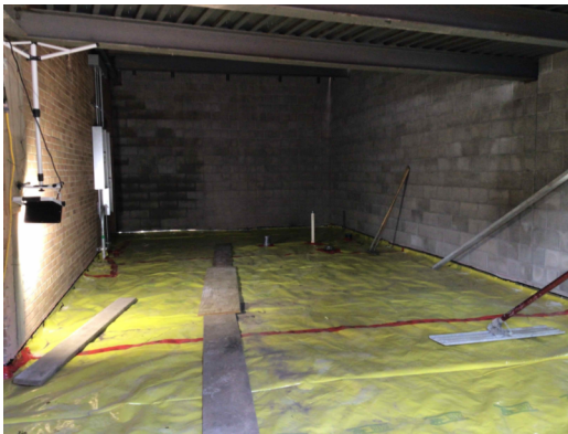
Sheridan Hills – Underground plumbing in the Kitchen.
